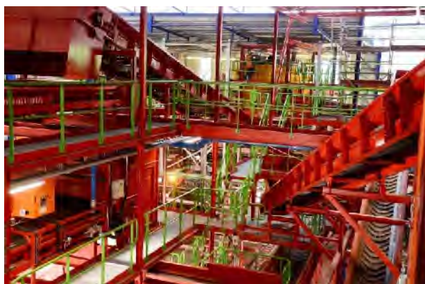
2014: Sorting plant for 80 kton post-separated and source-separated packaging waste
