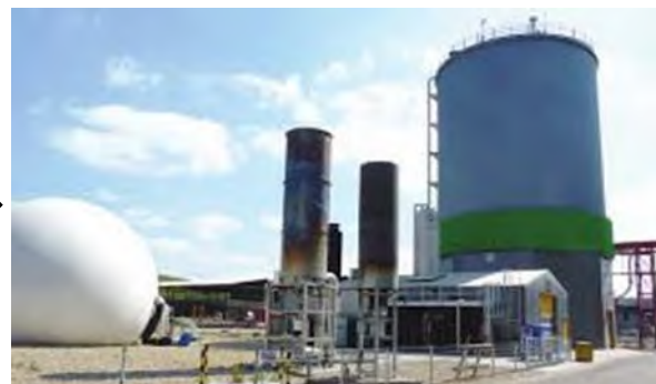
2012: Anaerobic digester for post-separated biowaste
