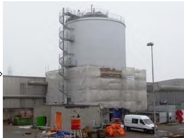
2013: Anaerobic digester for source-separated biowaste
